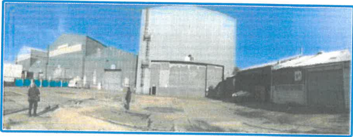
Rear of Unit 5
